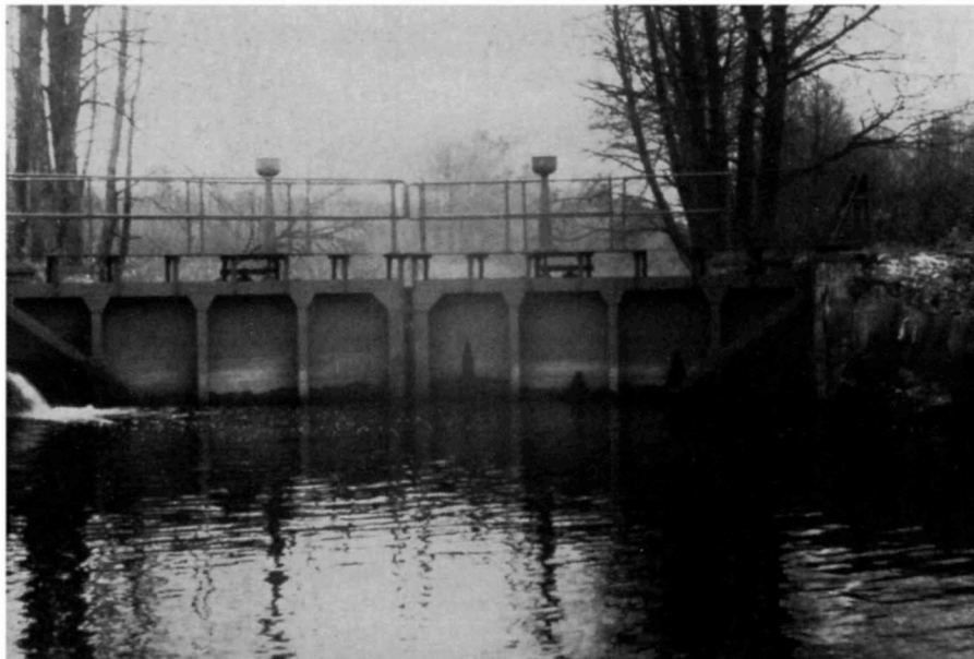
The bridge over the canal
